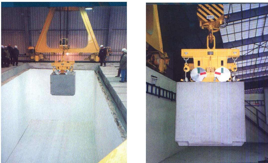
Fig. 3. Manipulation of the container during the process of its placing into the chamber of storage place.
