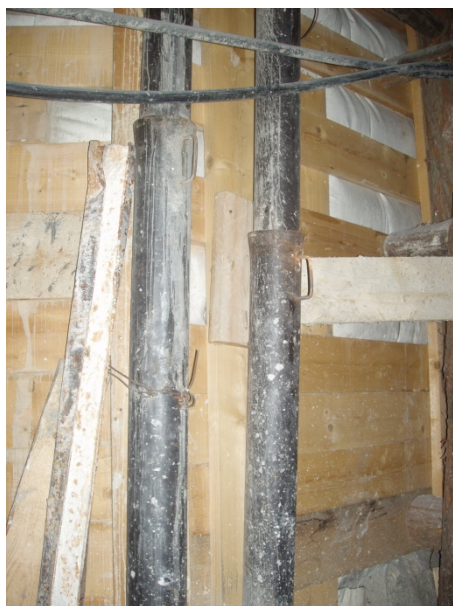
Fig. 8. Two-segment steel pipes.
