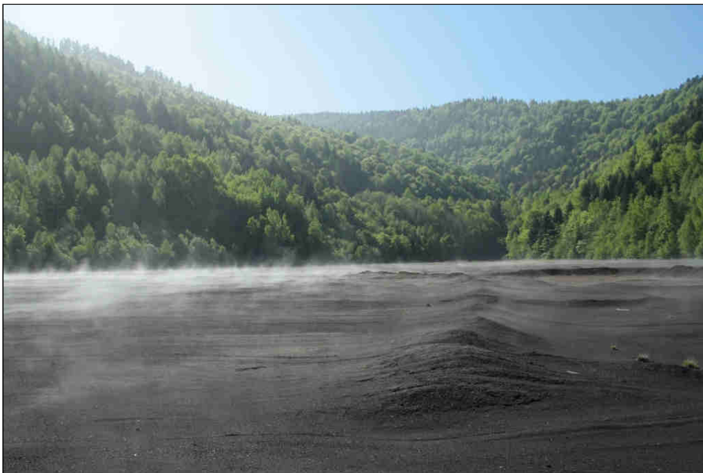
Fig. 7. The surface of Slovinky tailing impoundment (photo: authors).
