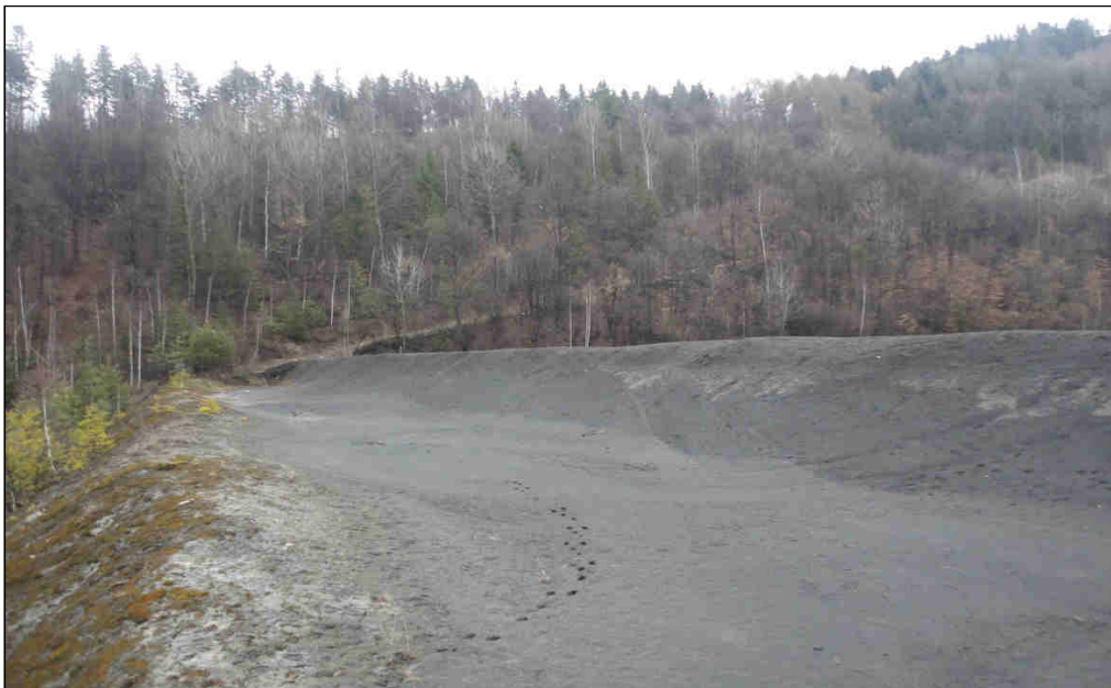
Fig. 6. The upper dyke of Slovinky tailing impoundment (photo: authors).
