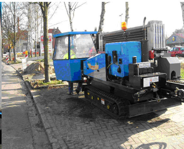
Fig. 4. Grundodrill 13 X over-boring a 60 kV cable.
