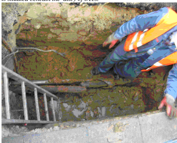
Fig. 5. Threading the bore head into a new wash over section.
