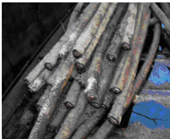
Fig. 6. The recovered old 60 kV cable inside the transport container.
