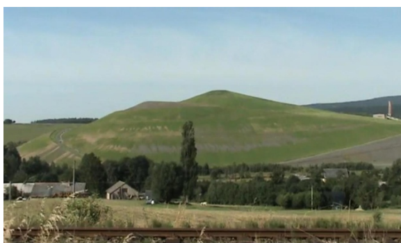
Fig. 10. Central Heap after grassing, July 2009 [1].
