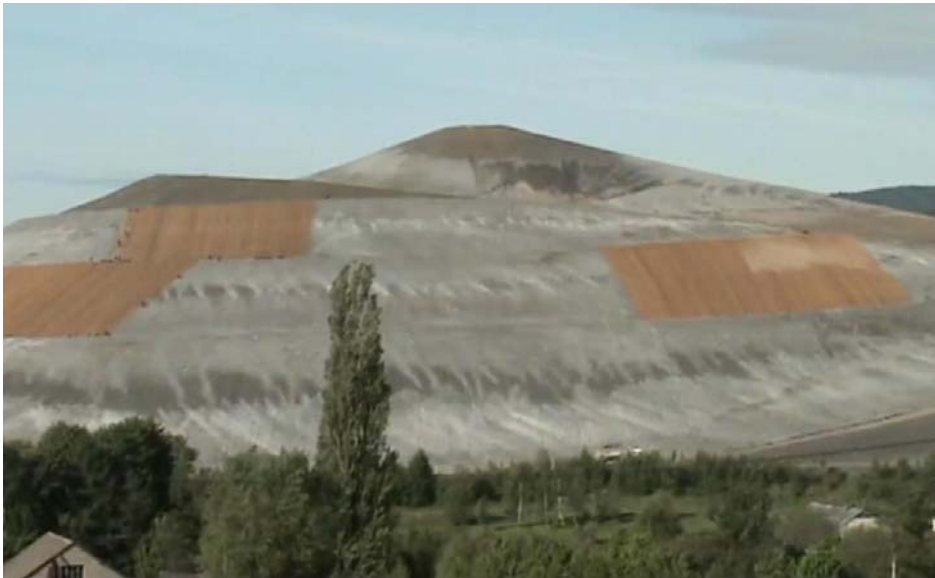
Fig. 6. Central Heap after hydroseeding and coconut mats [1].
