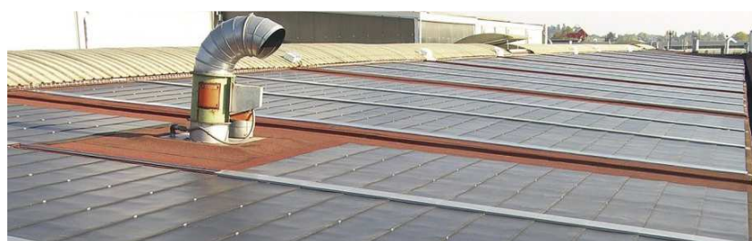
Fig. 3. Roof with PV system Tegola Solar (Ušák, 2014).
