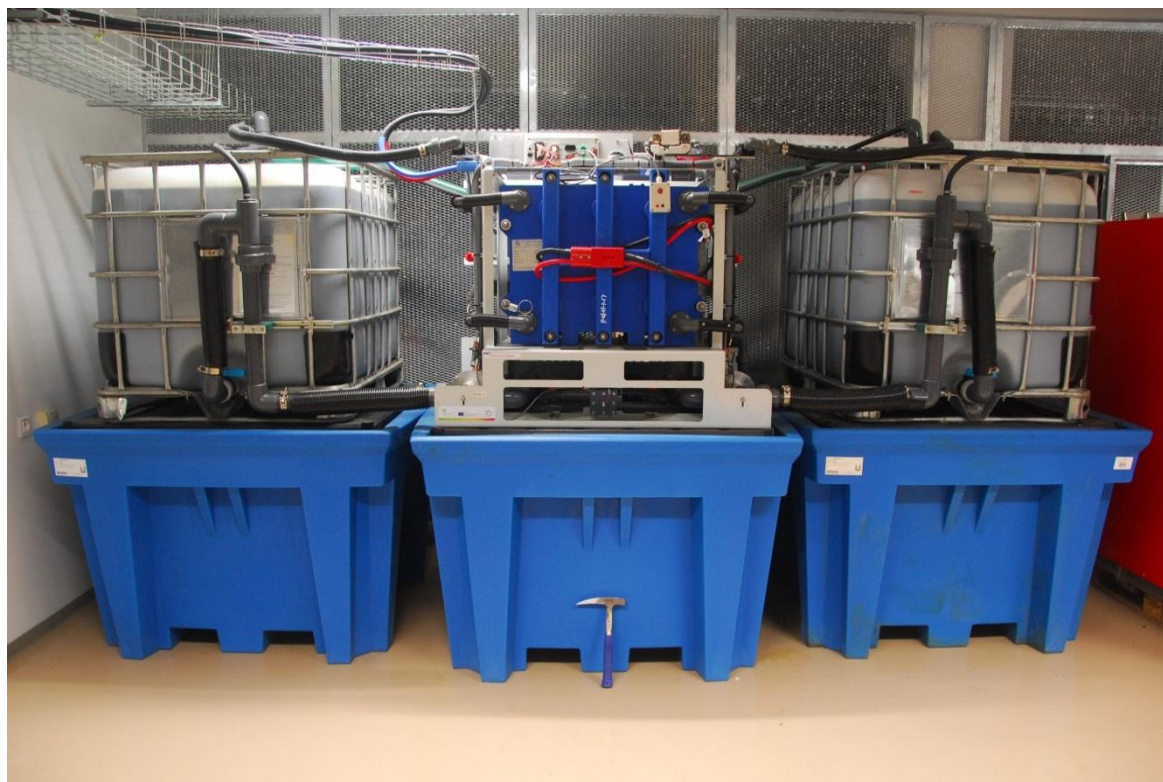
Fig. 2. An actual commercial vanadium flow cell. The left and right upper containers in the transport cages hold the respective vanadium solutions. The middle is the armature of the electrochemical cell. The containers and the cell are placed over the blue reservoirs intended to capture any spill in case of an accident. For sizing an Estwing 22, a 13" geological hammer, is leaning against the middle retention reservoir.
