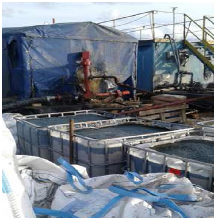
Fig. 2. Insulating compound ready for injection
