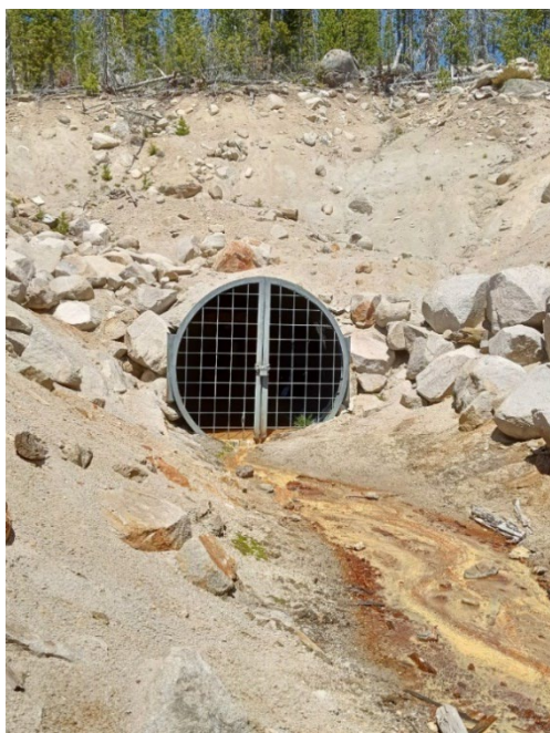
Figure 4 Discharge of acid mine drainage water from the Crystal mine
