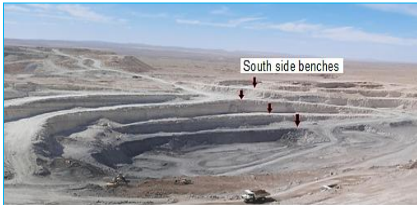
Fig. 4. Slopes on the south side of the Northwest block
