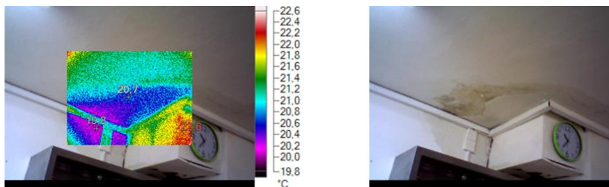
Fig.5 The part of the ceiling and cabinets where water seeps in Source: Begáni, 2021
