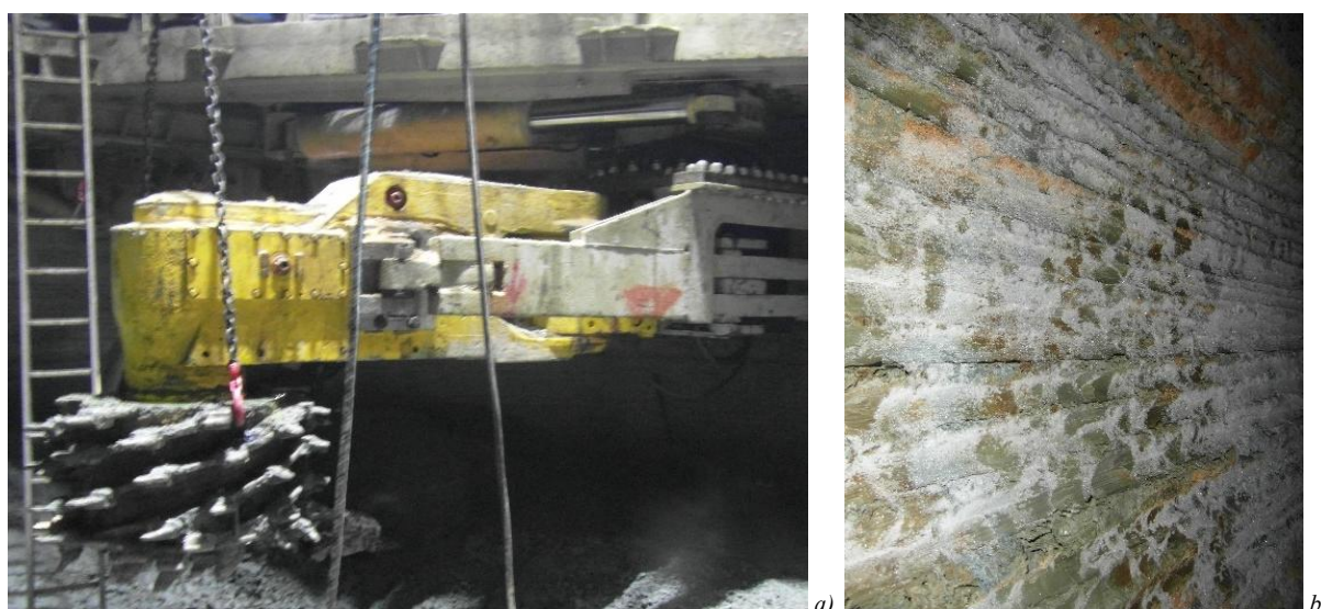
Fig. 7. Excavation of shaft GG-1 (Boloż, 2025): a). KDS-2 machine, b). side wall with visible frost made with the cutting head
