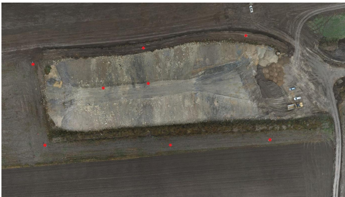
Fig. 4 Positions of the Emesent Hovermap ST-X GCPs (red dots, highly reflective targets – see Fig. 2e)
