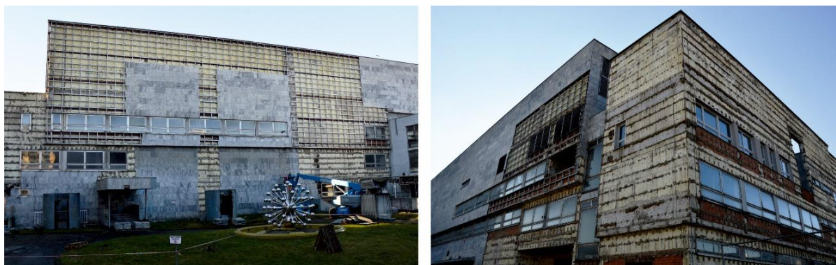
Fig. 2. Removal of the marble cladding from the Istropolis building (photo: Ružička, February 2022)
